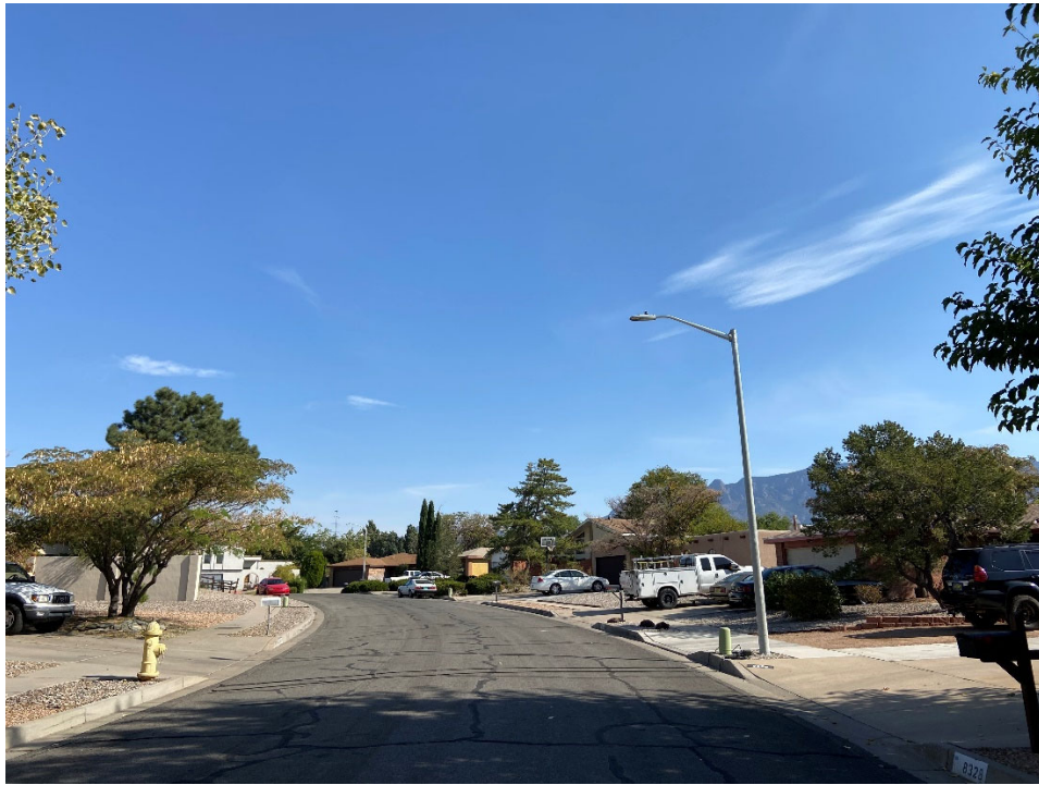
Figure 3: Ruidoso Road looking Northwest
